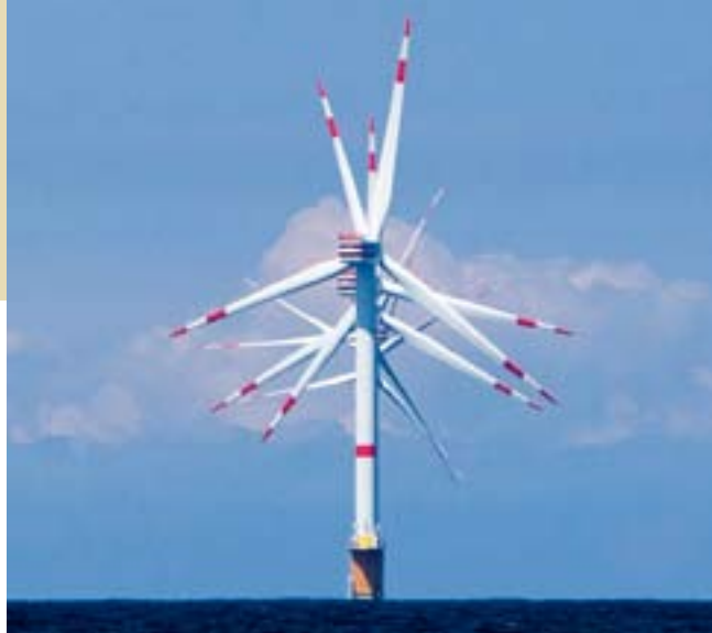
Thornton bank, Ostend, Belgium © EWEA
