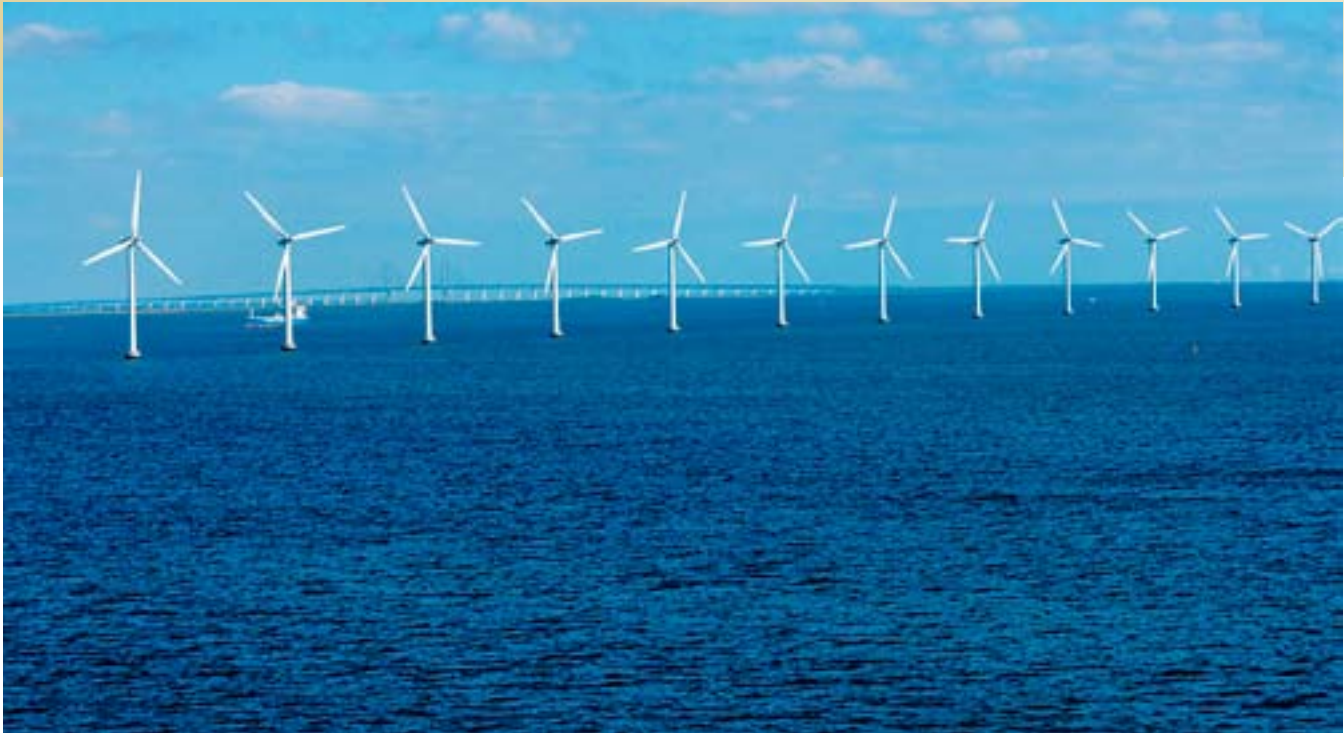
Offshore wind farm in Baltic Sea off Copenhagen, Denmark © Tony Moran
