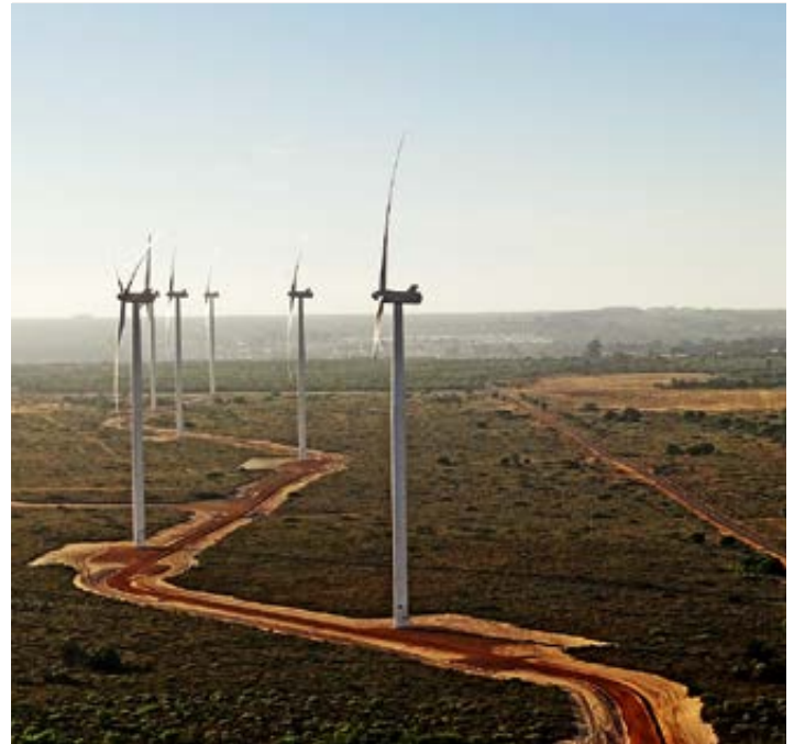
Hopefield Wind Farm © Umoya Energy
