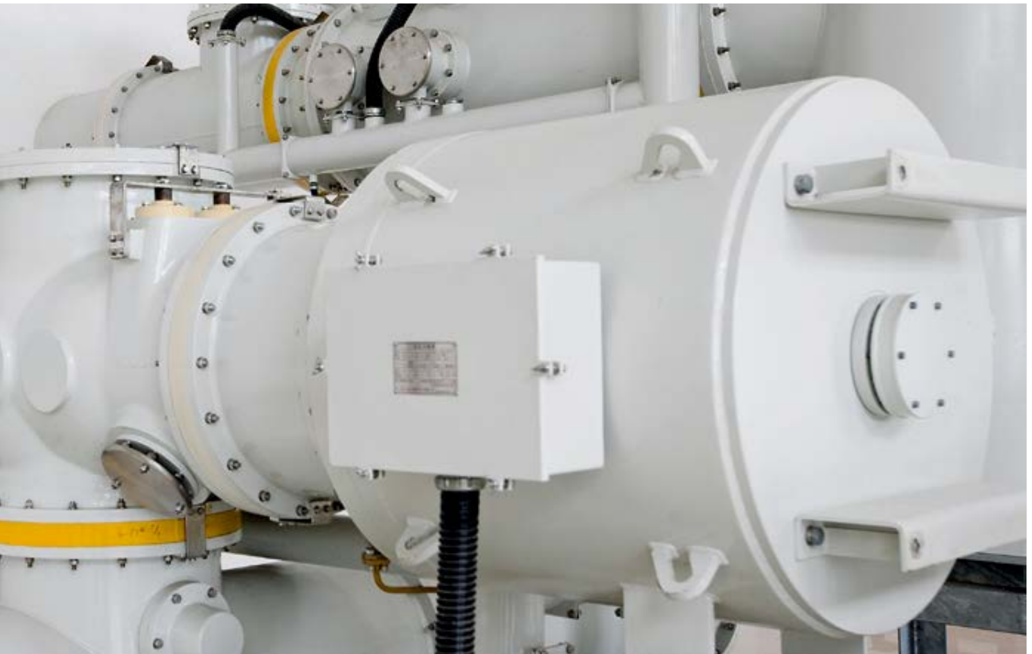
© Wind Power Works
