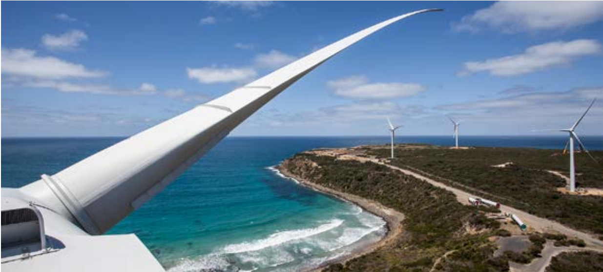
Portland wind farm © Pacific Hydro
